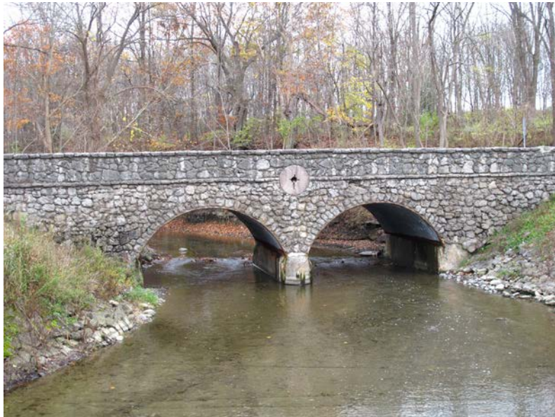
Papermill Park Bridge (Town of Avon)
