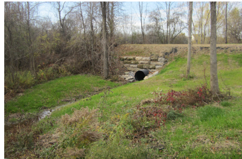
The GVC helped to repair the Railroad Bed Trail in Avon after a significant flooding event in 2015 (Photo: GVC)
