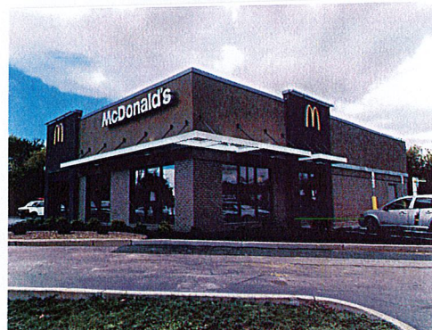
Side entrance to lobby, aluminum trellis. Existing building built in 1994.
