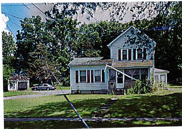
Purchased by Unknown Investment Firm garage and shed being demolished
